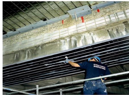
At site level, prior to the installation of carbon fibre plates, the concrete surface must be prepared to remove the laitance by either grit blasting, needle gunning or planing, followed by vacuum cleaning to remove any dust. At this point the concrete may be tested for adhesion.
