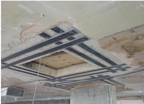
Composites come in a variety of materials, each having its own unique property – carbon fibre, aramid fibre and glass fibre.
