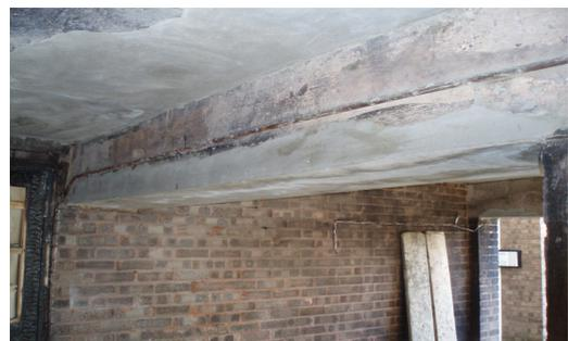
Furthermore the concrete can be enhanced using specialist stain and smoke covering coatings or pigmented anti-carbonation coatings.
