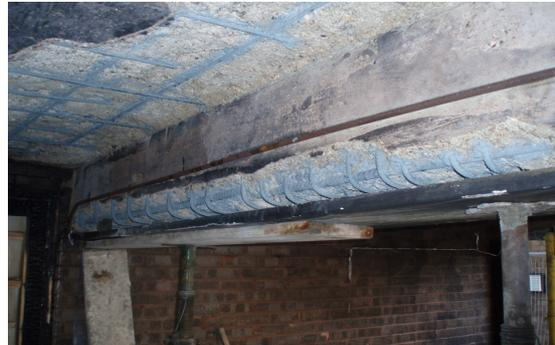
The repair of the structure begins with a visual survey and hammer test of the concrete elements. This establishes the extent of pink concrete as well as hollow and defective areas.
