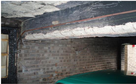
The residual strength of structural-quality concrete exposed to fires of up to 300°C is not severely reduced. Concrete exposed to temperatures greater than 500°C can have its compressive strength reduced significantly and advice may be required from a structural engineer.
